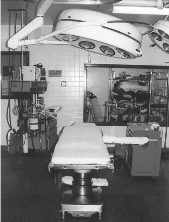
Figure 89-3 Typical OR layout showing OR table, overhead lights, anesthesia machine and monitors, medication and supplies cart, storage room, and wall outlets for gases.
